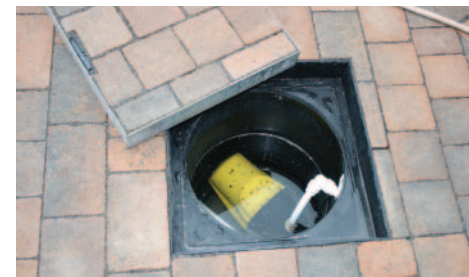
The Aquaflow® permeable paving system allows filtered water to be stored and then pumped back for secondary use.
