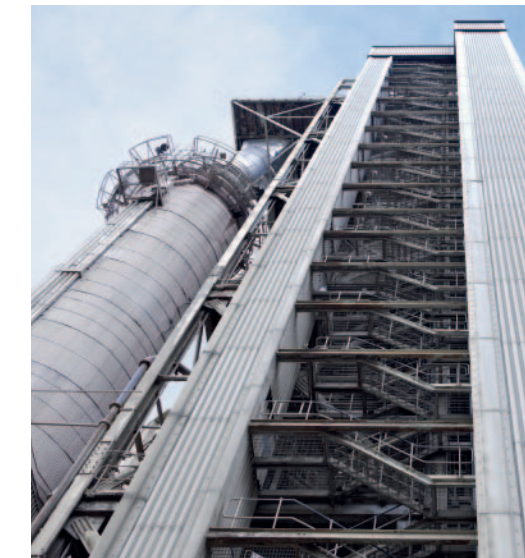
Ketton cement works.
