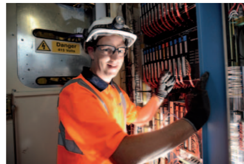
Electrical supervisor James Veakins reduced lighting costs by 75% by improving control systems at Whatley quarry.
