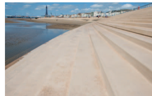
GGBS was used in the concrete for new sea defences at Blackpool, Lancashire.
