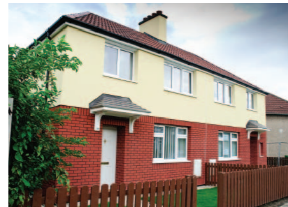
Before and after... an award-winning regeneration scheme in Liverpool used Hanson Structherm's cladding systems
