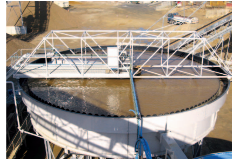
The new marine sand and gravel processing plant at Frindsbury Wharf on the river Medway features an enclosed water recycling plant
