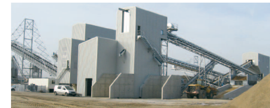
A new £3.6 million marine sand and gravel processing plant at Frindsbury Wharf on the river Medway in Kent is fitted with metering equipment to allow specific energy consumption data to be produced and interrogated
